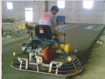
[ Working to get that superflat warehouse floor. ]
