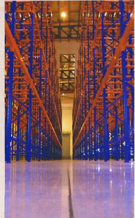
[ Special floor finishing techniques were applied on the Sankyu warehouse concrete floor to produce a smooth, highly reflective finish. ]
